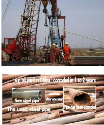
Fig. 10 The steel pipe corrosion due to water injection into the oil layer.
