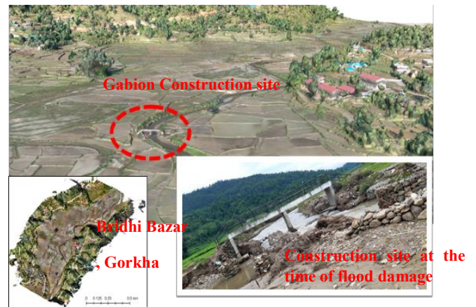
Figure 1 : The location of the construction site
