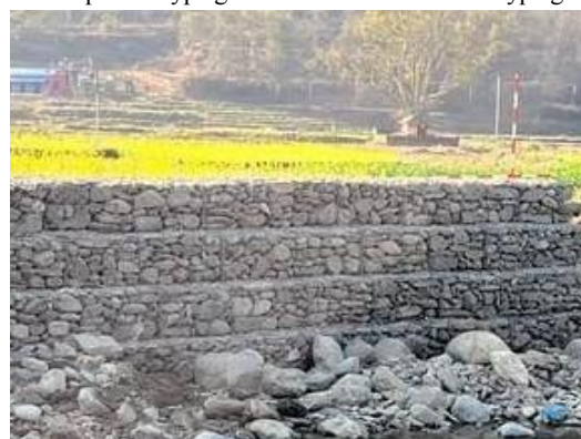
Picture 1: Japanese Type Gabion constructed at site
