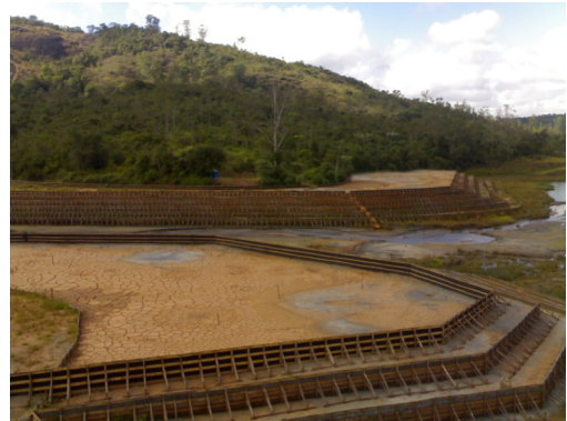
Figure 3.23. Geotubes as structural elements in upstream method phosphate tailings dams (Gomes, 2007).
