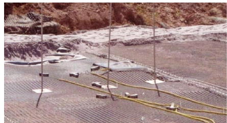
Figure 2.12–Instruments on site (Spotti,2006)
