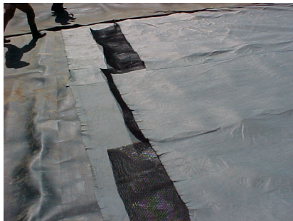
Figure 4.2: Example of liner used in MSW landfill in Brazil. (a) cross section; (b) HDPE geomembrane and drainage geocomposite deployment (Vidal, 2003).
