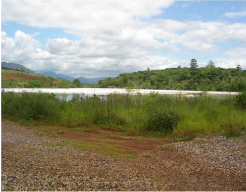
Figure 3.21. Phosphate tailings lagoon: general view
