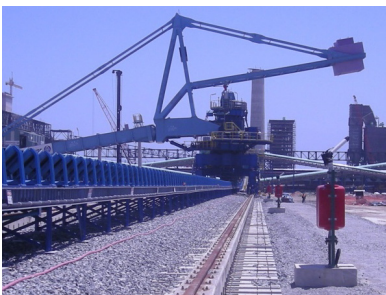
Figure 2.30- Stacking machine fill on GECs
