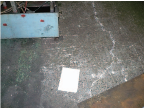
Fig. 6 The trace on the concrete floor by displacement of a manufacturing machine shown at the upper left part and the cracked floor. White rectangular is 257 x 182 mm notebook.
