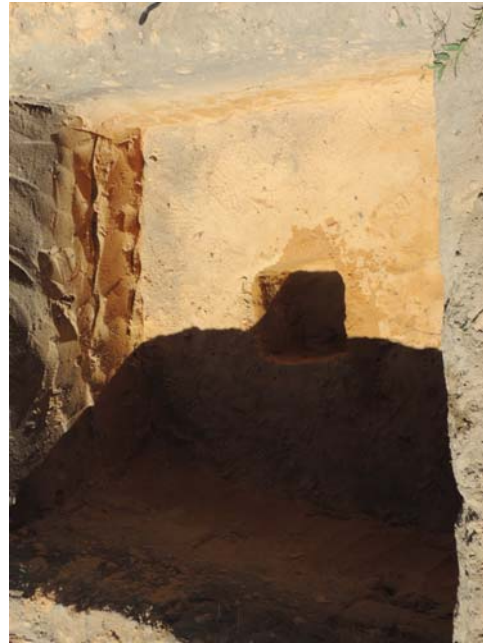
Figure 18. Detail of Excavation and Hole for Permeability Testing
