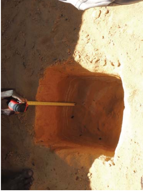
Figure 15. Pre-soaking the hole
