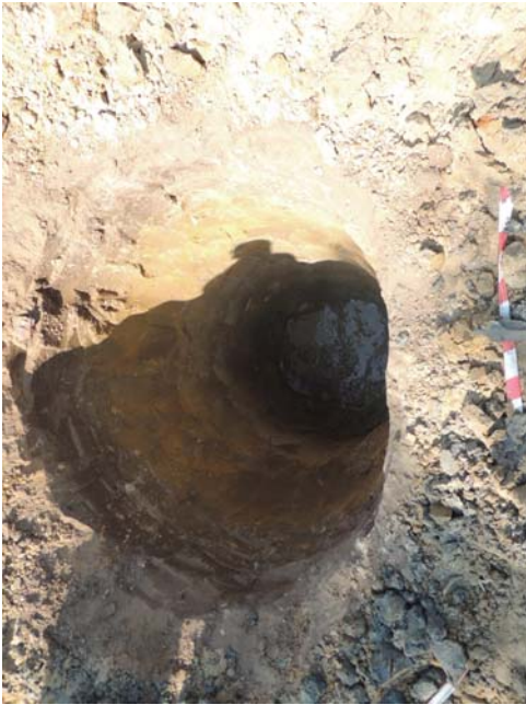
Figure 11. Excavation of Trial Pit, sampling at 1.75m
