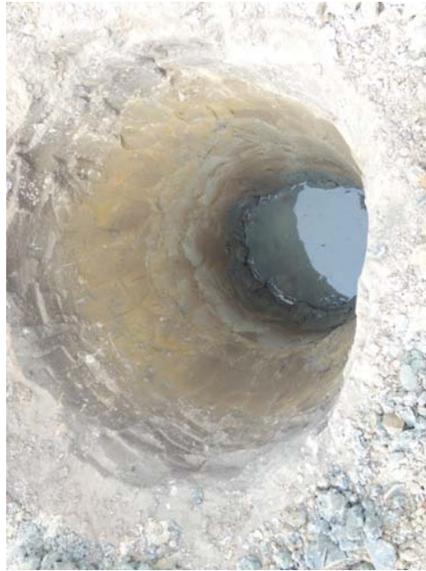
Figure 12. Excavation of Trial Pit, water table at 2.0m
