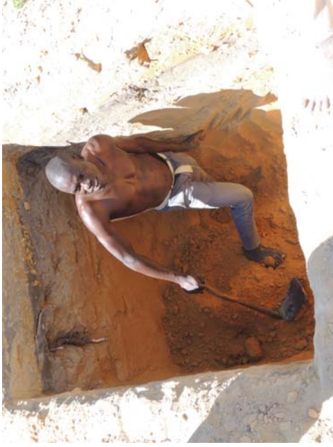
Figure 11. Excavation of Trial Pit, sampling at 1.75m
