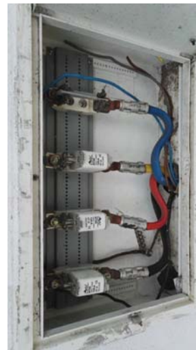
Figure 19. Connectors to the MDB
