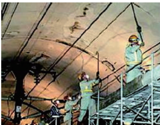
Fig.2 Hammering - usual procedure of tunnel inspection (Mainichi news paper)
