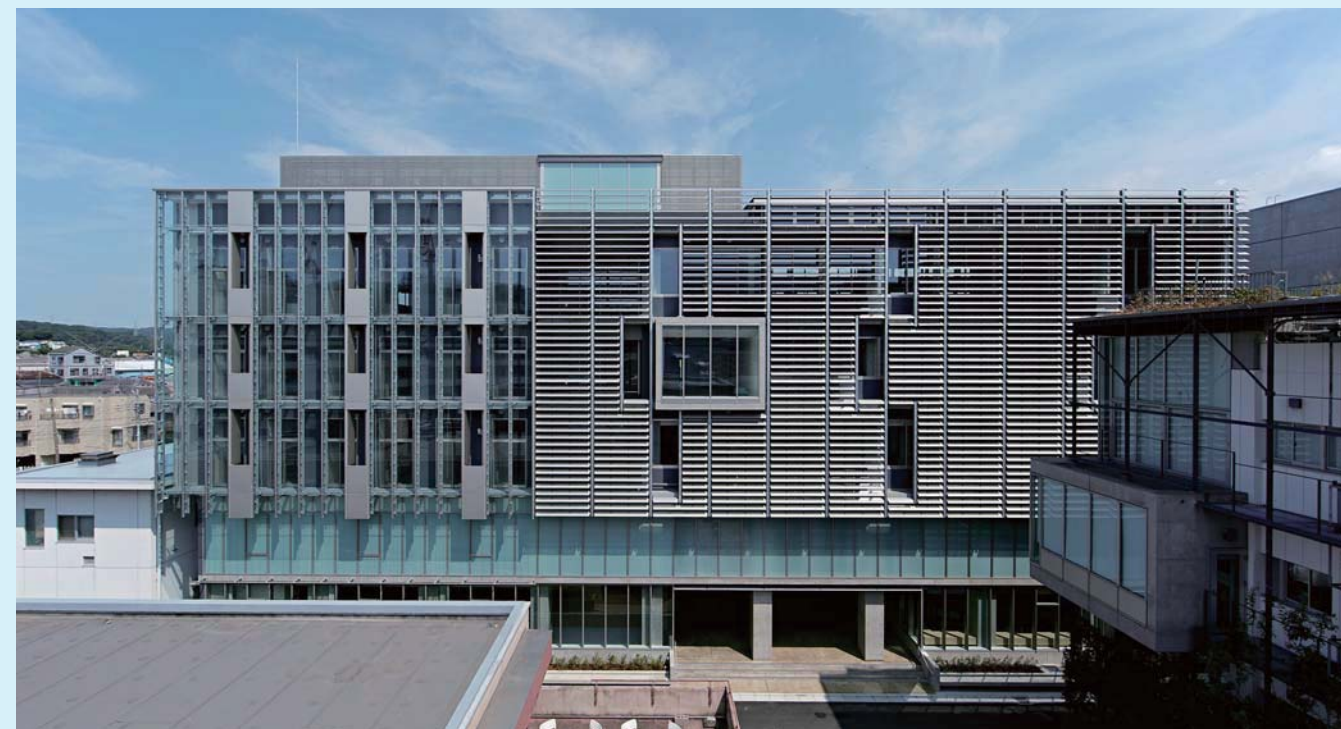
建物南東面のファサード | South East Facade
