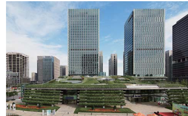
TEDA MSD Complex (Tianjin, China)
