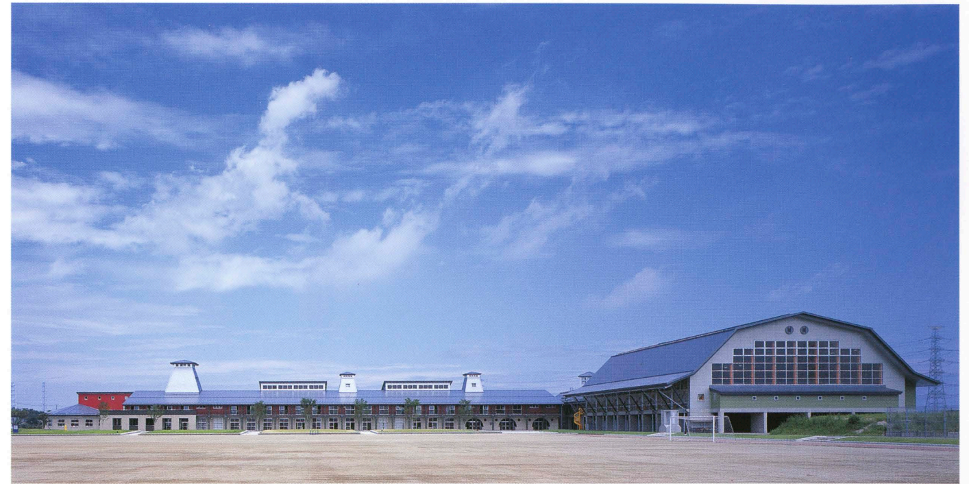
グラウンド側全景 General view from the school ground.
