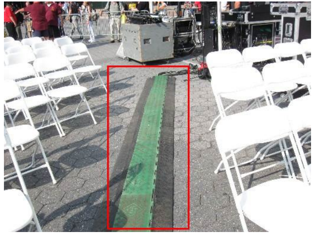
The area should be clean, orderly. The electric wires should be secured by cord covers in order to minimize the tripping hazards.
