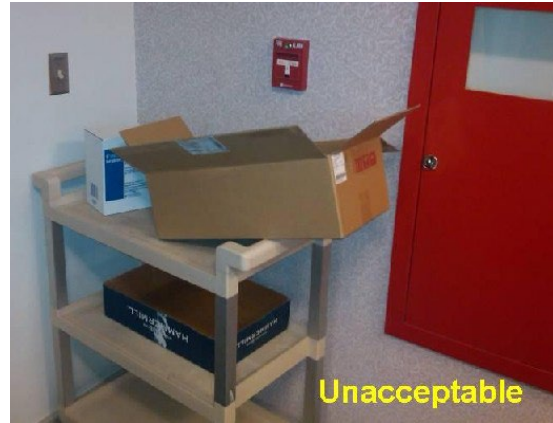
Obstructed Manual Pull Station
