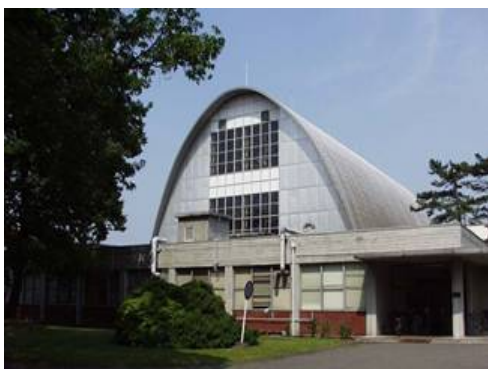
Gamma-ray irradiation facility building
