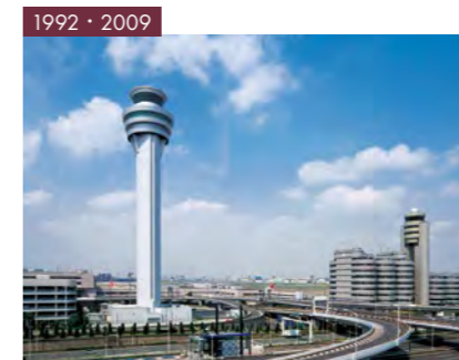
東京国際空港（羽田）庁舎・管制塔 Tokyo International Airport (Haneda) Administration Office Building and Control Tower
